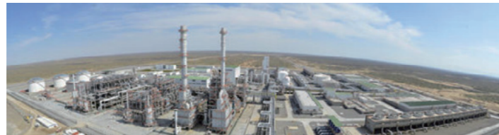
Gas-to-gasoline (GTG) plant
