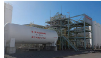
Liquefaction system using the new type of hydrogen liquefier
