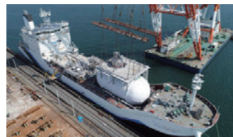
Installation of liquefied hydrogen tank for marine transport
