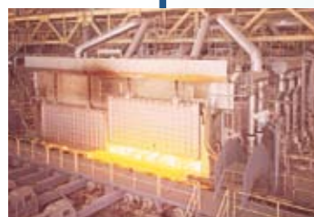
製鉄用油圧装置 Hydraulic equipment for steel making plant
