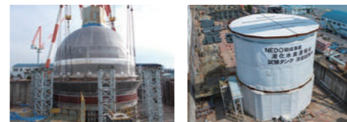
Establishment of tank manufacturing technology and structural analysis technology A 40,000 m 3 class test tank
