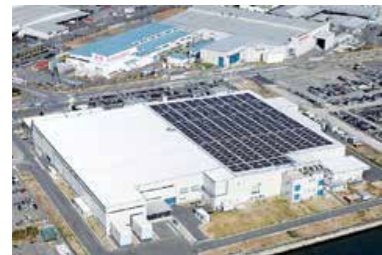
Figure 13: Nagoya Works 1: 750-kW power generation facility
