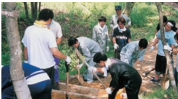
Volunteers building a trail (chip road)
